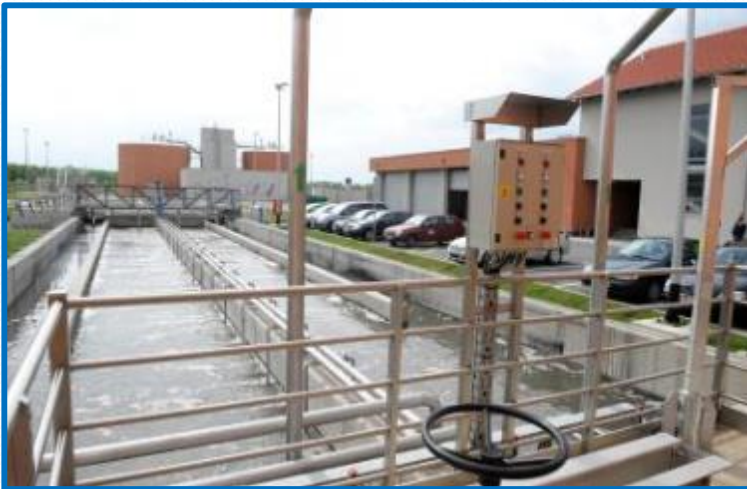
Wastewater treatment plant in Croatia, financed with the help of EU funds
